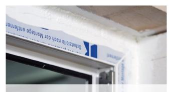
PU Safe forms a thin, rainwater-proof and flexible membrane that adheres well to all conventional materials.
